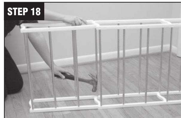
STEP 18: Tap connections together as shown, on a firm surface only.
